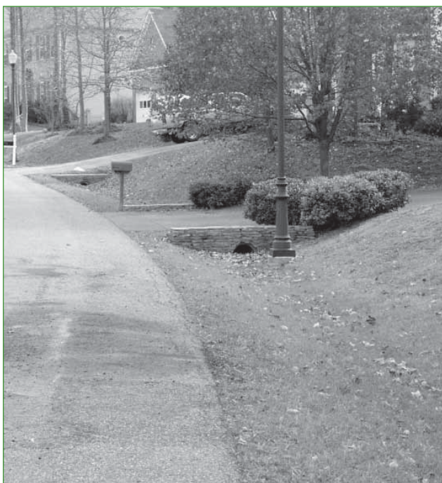
Vegetated open channel along residential street
